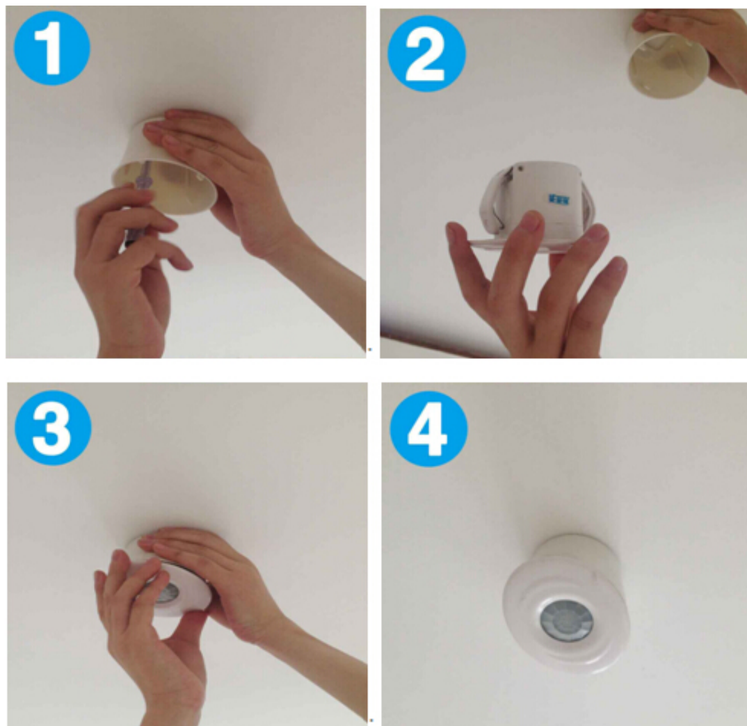
Fig. 4 Installation with a Holder
