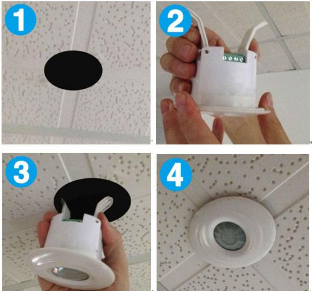
Fig. 5 Installation without a Holder
